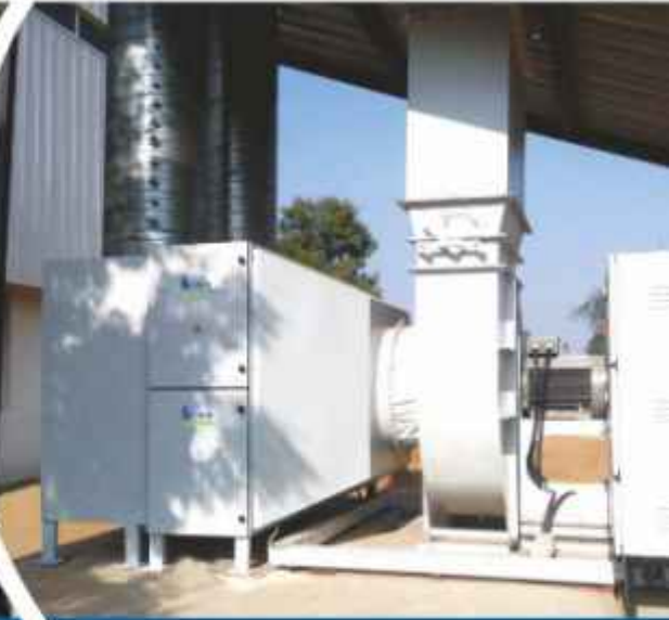
Outdoor installation of fume extraction system
